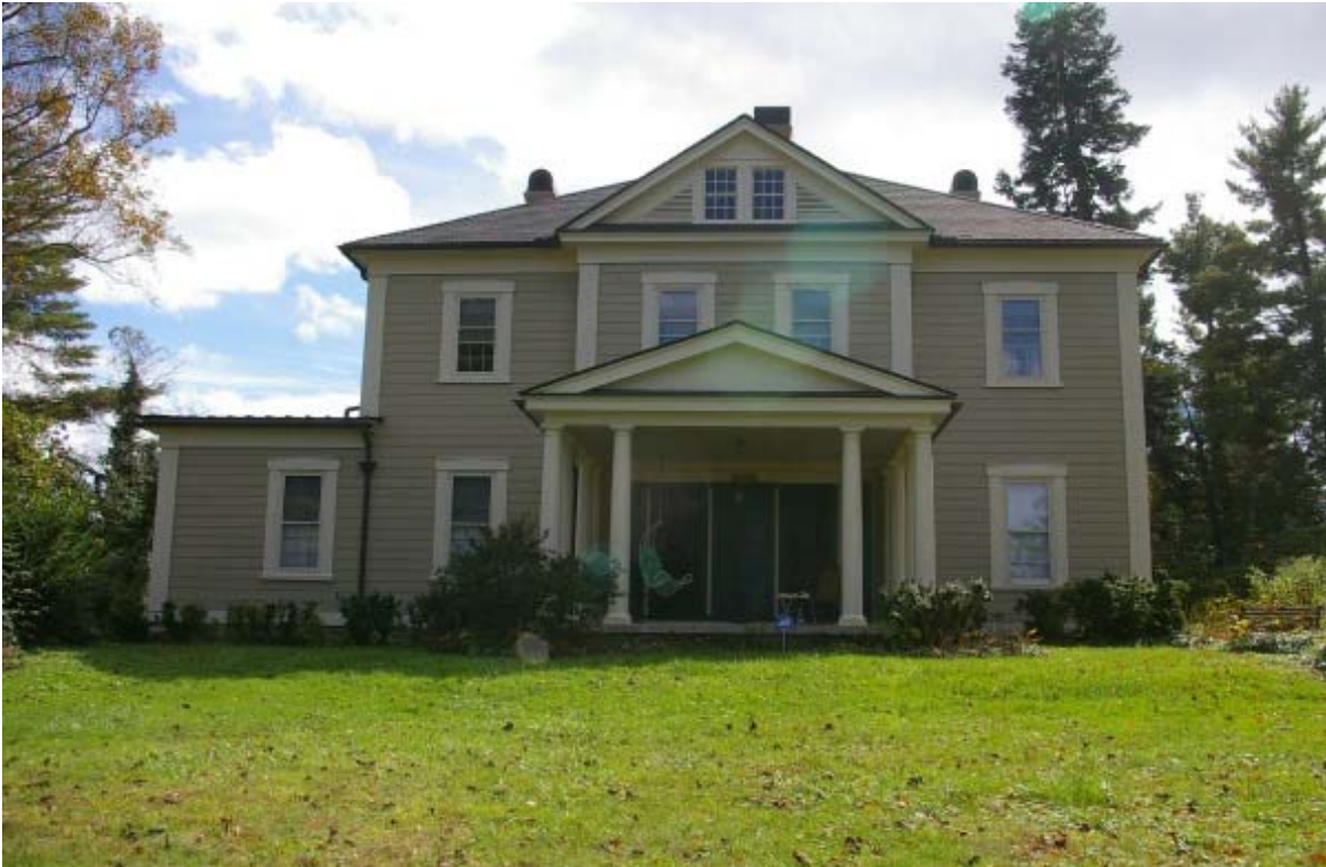
3. North elevation, view S
