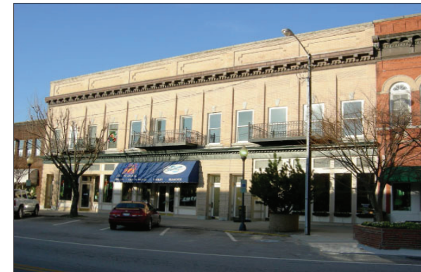
503-511 North Main Street before and after rehabilitated facade.
